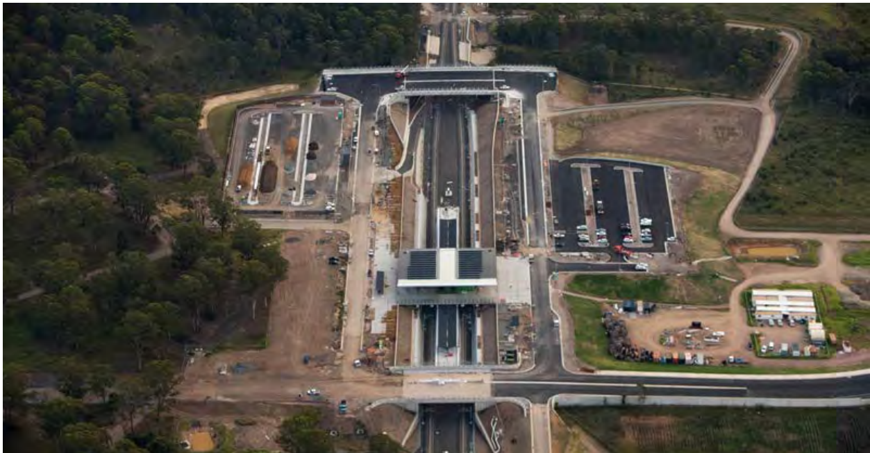
Figure 5-5 Edmondson Park Station
